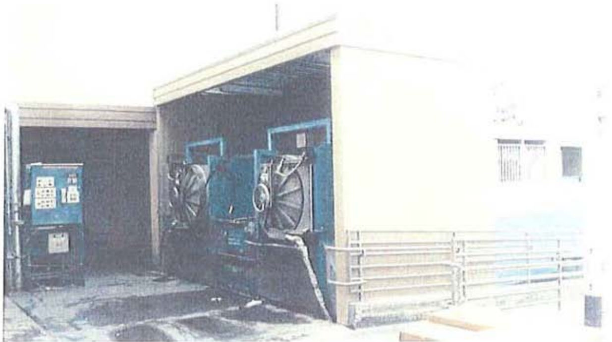
Mitigation Measure 3.4-6 – Trash Compactor Enclosure with Sound Absorption Panels (Back View)
