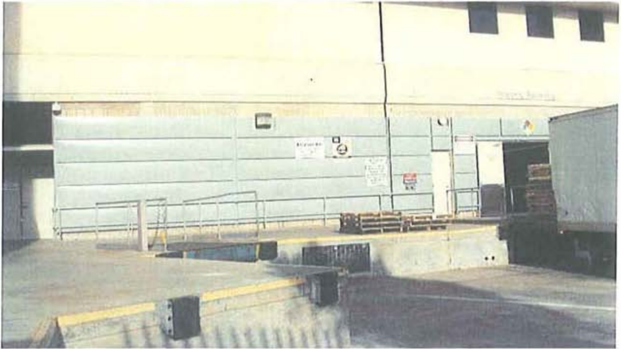
Mitigation Measure 3.4-5 – Loading Dock Sound Absorption Panels
