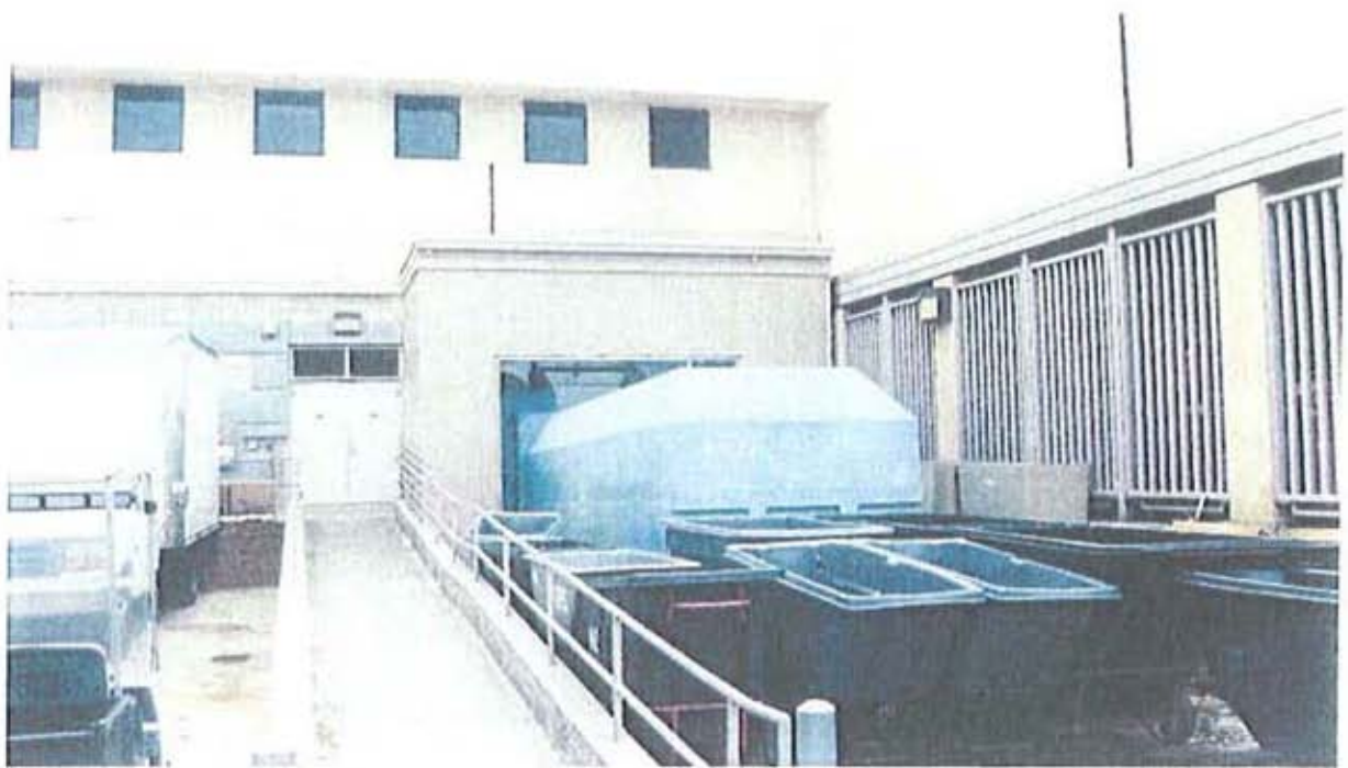
Mitigation Measure 3.4-6 – Trash Compactor Enclosure with Sound Absorption Panels (Front View)
