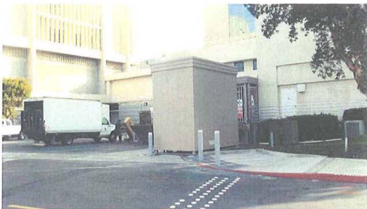
Mitigation Measure 3.4-6 – Baler Enclosure with Sound Absorption Panels
